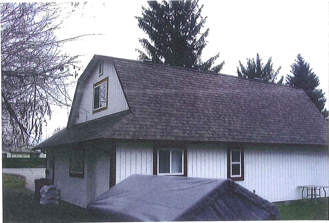
BACK OF #2085-2 FROM LOT CORNER
