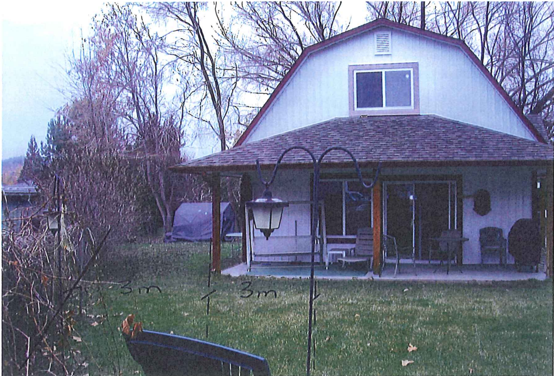
SOUTH SIDE VIEW OF # 2085-2 WITH REAR YARD (PROPOSED 3m REAR YARD VARIANCE.)
